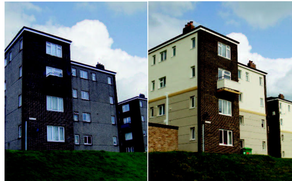
External improvements to Sowerby Road
